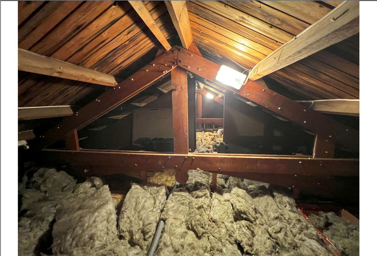
Building 1 Roof Structure
