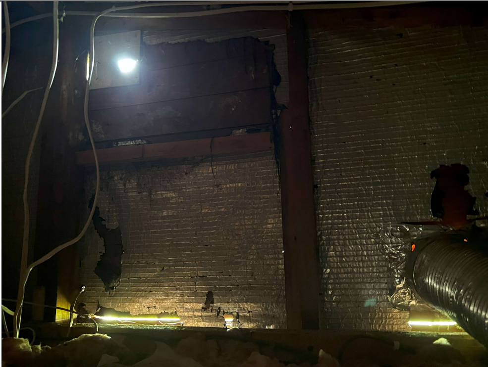
Building 3 Gable End
