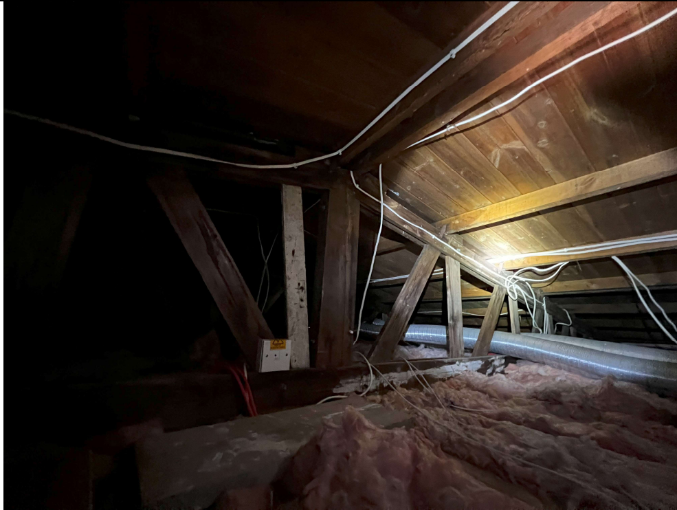
Building 3 Roof Space
